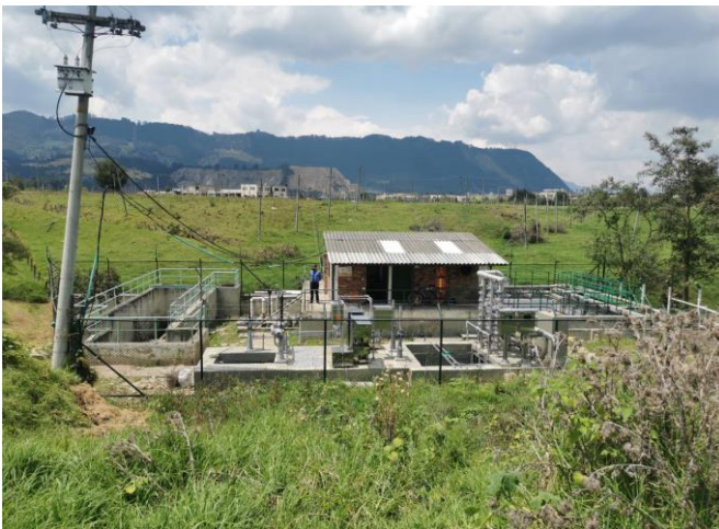
PTAR Rincón Santo
