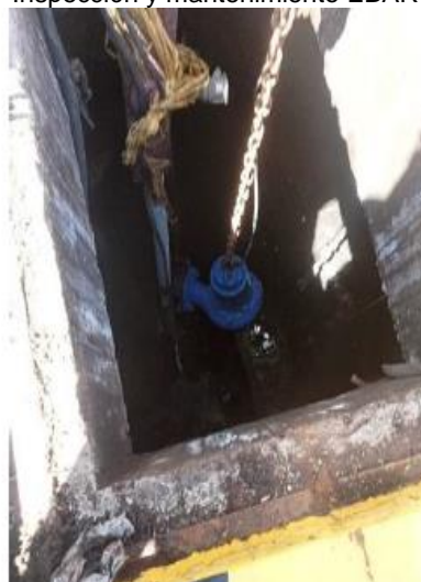
Electrobombas sumergibles
