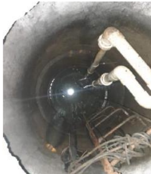
Electrobombas sumergibles
